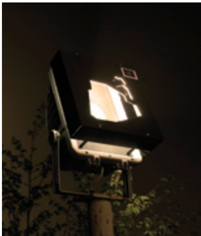
Nature-friendlier lamp (left) which enables shading of the flight openings for bats at the belfry and above church doors (right)
