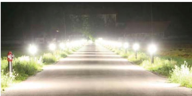
Access road to the cultural monument. This is an example of senseless and harmful investment: unbearable glare, light shining above the horizontal, and high maintenance costs. Also, the lawn around the luminaires will require manual mowing.
