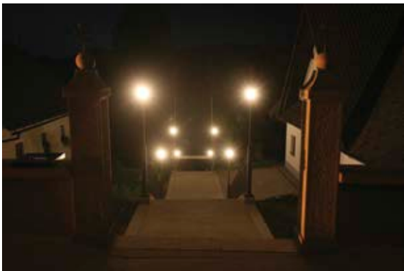
Entry into the church with unshielded lamps on short poles shining into people's eyes from the direct vicinity. We should use fully shielded lamps even if the legislation does not require it.
